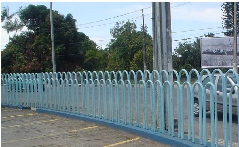
Figura 90 ó Gradil do Shopping Grê-Center.
